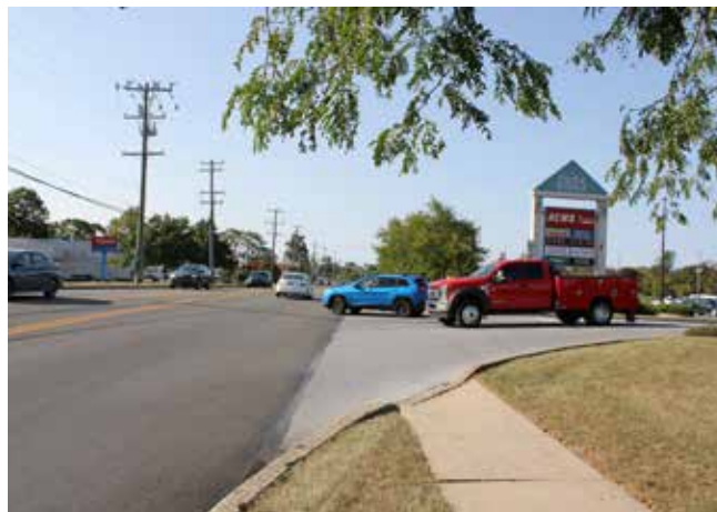
This entrance to Park Ridge Shopping Center is an example of an older driveway design that could be enhanced to reduce the possibility of vehicle conflicts and improve safety for pedestrians.
